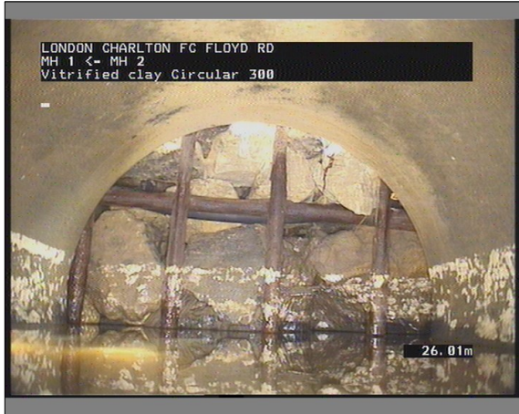
Photo: 1_1_3_A.JPG 26.01m, Finish node type, manhole reference number: U/S
