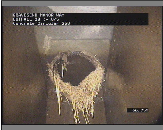
Photo: 5_5_12_A.JPG 66.95m, Finish node type, manhole reference number: U/S
